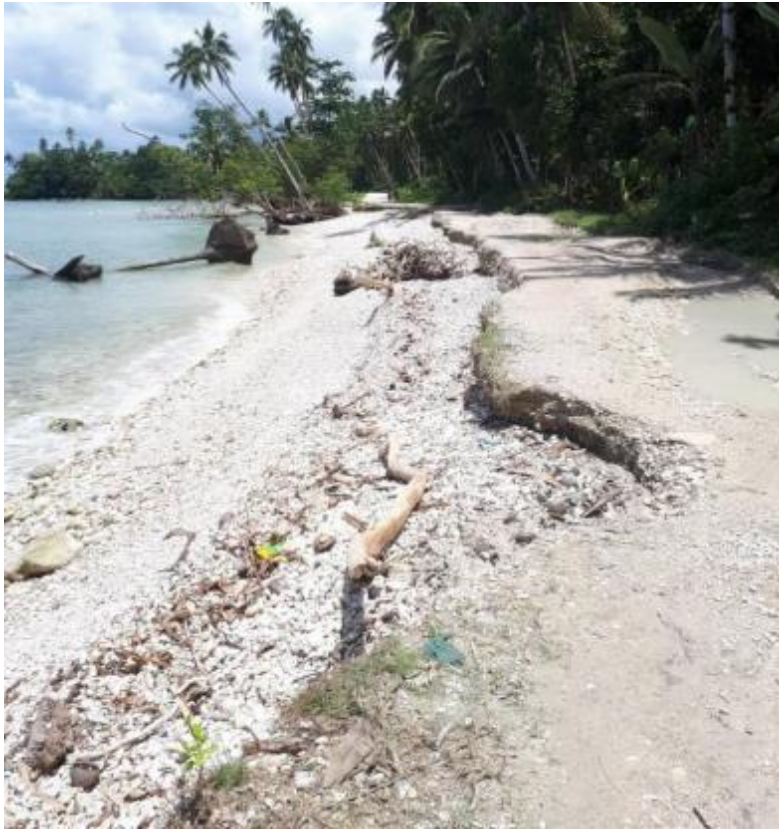
Figure 11: Road erosion along coastline on northern road
