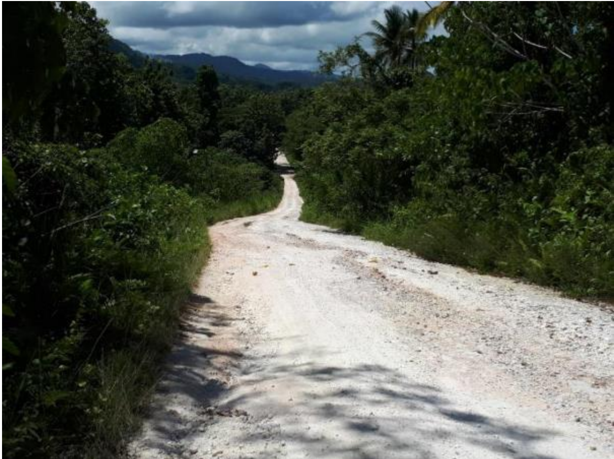
Figure 14: Steep section on southern road showing signs of run off and gullies.
